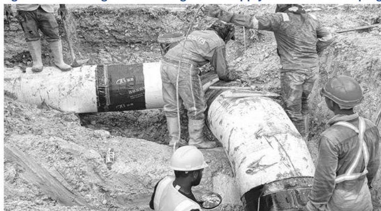
Figure 9: Trenching and Installing Water Supply Infrastructure Piping
