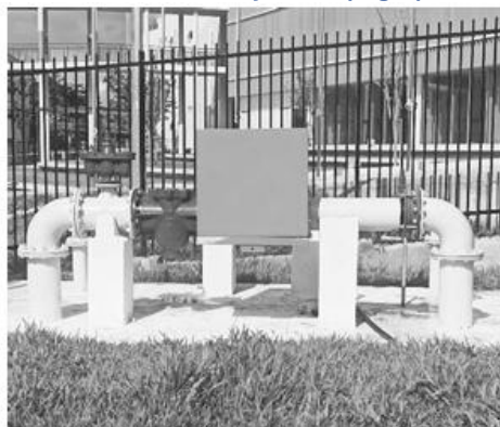
Figure 6: Construction and Installation of Piping Systems Featuring Metering Point (left) and Cold and Hot Water Systems (Right)
