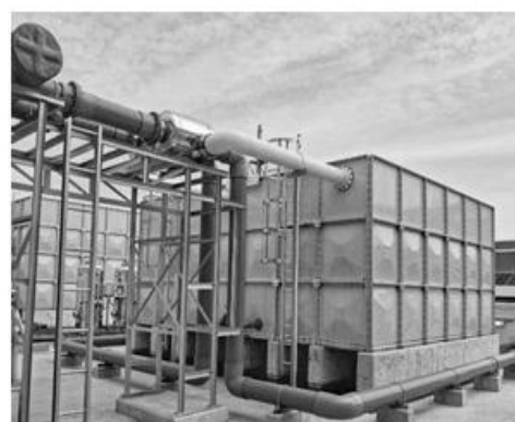
Figure 7: Value-added Components Featuring Oil Separator (left) and Rainwater Harvesting System (Right)
